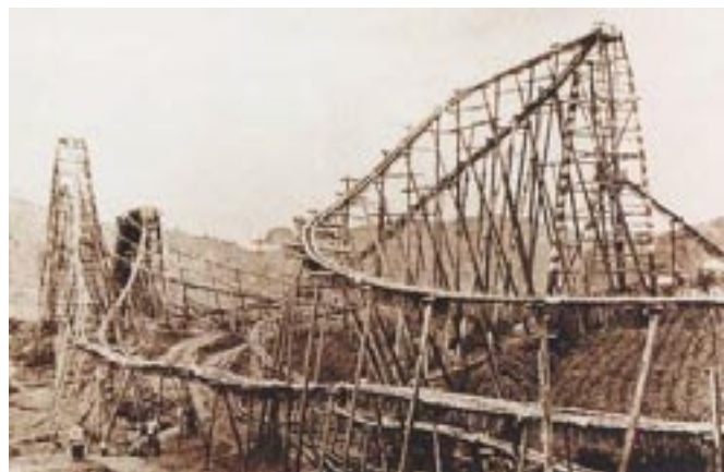
Figure 12. Gravity driven bamboo pipelines. Note water-lifting system on right.
