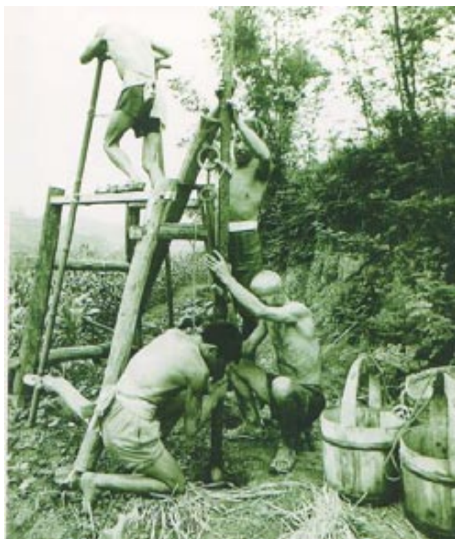
Figure 4. A modern recreation of drilling technique from the North Song Dynasty (960-1127 AD).
