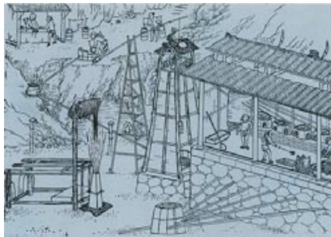
Figure 13. An ancient sketch originally from "The Annals of Salt Law of Sichuan Province". A "Kang Pen" drum is seen in the centre foreground, with gas pipes directly feeding the salt stoves on the right. At the top, brine from a remote well is being carried in buckets by men, who feed it into a bamboo pipeline that runs down to the stoves. One of the carriers is being paid at top left, and it appears that a blow out is depicted on a new well being drilled in the left foreground; maybe the men operating the drill rig have run away, as tragically happened at a Chongqing, Sichuan sour gas well, late 2003.
