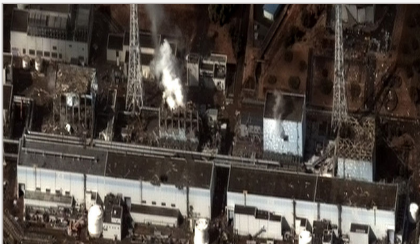
The damaged Fukushima I Nuclear Power Plant after the 2011 Tohoku earthquake and tsunami. (Credit: Digital Globe)
