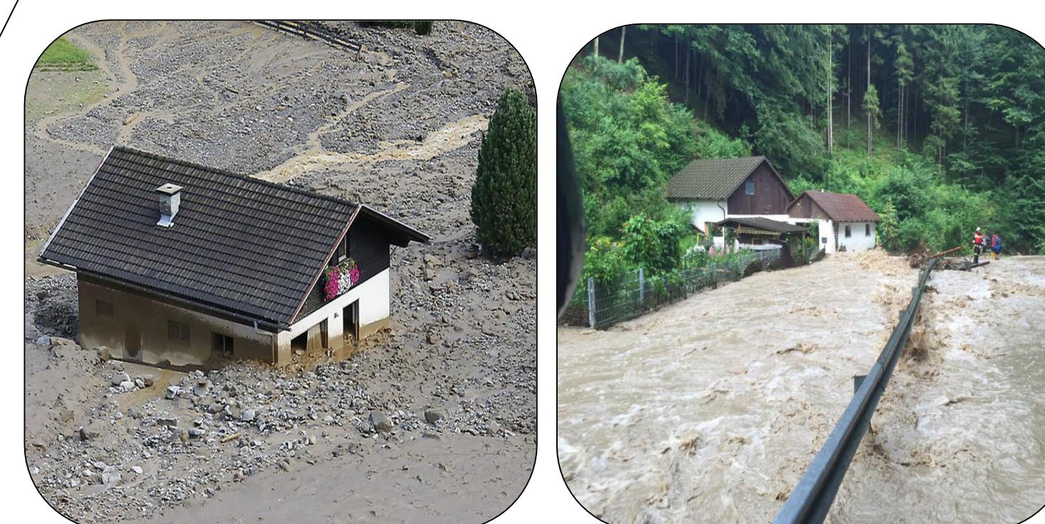
Debris flow Flood
