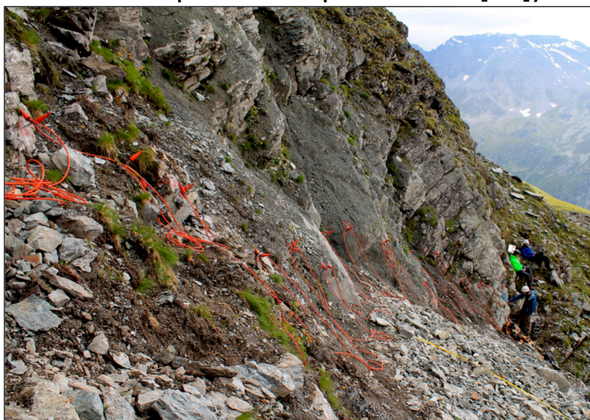
Fig. 9: Western part of rockwall 2 (S4).
