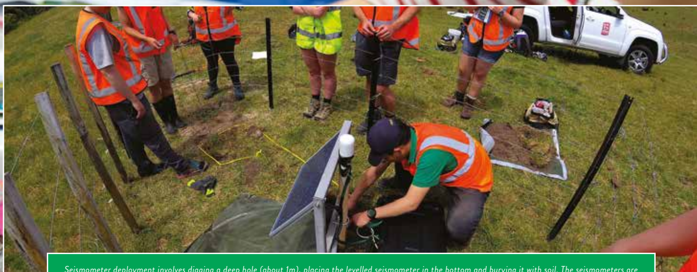
Seismometer deployment involves digging a deep hole (about 1m), placing the levelled seismometer in the bottom and burying it with soil. The seismometers are powered by solar panels, with a car battery for back-up. Sites are protected from animals with fences. Photo courtesy of Sian Evans.
