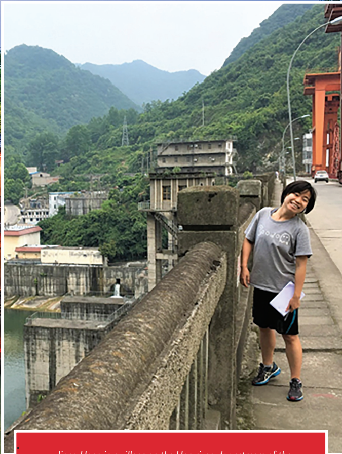
Jiang Hong in a village on the Han river, downstream of the Dankiangkou dam. Hong is a PhD student working on the project.
