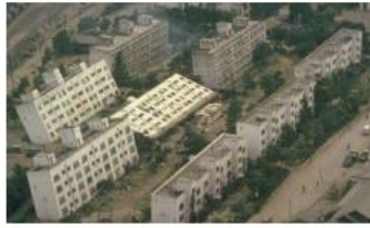
What earthquakes can do to buildings on soft ground
