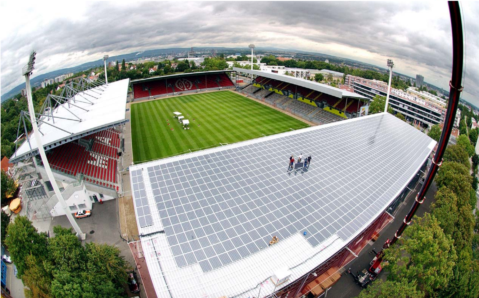
Soccer Stadium 1. FSV Mainz 05, Germany: 240.8 kWp (modules supplied by Sharp & S.E. Project)
