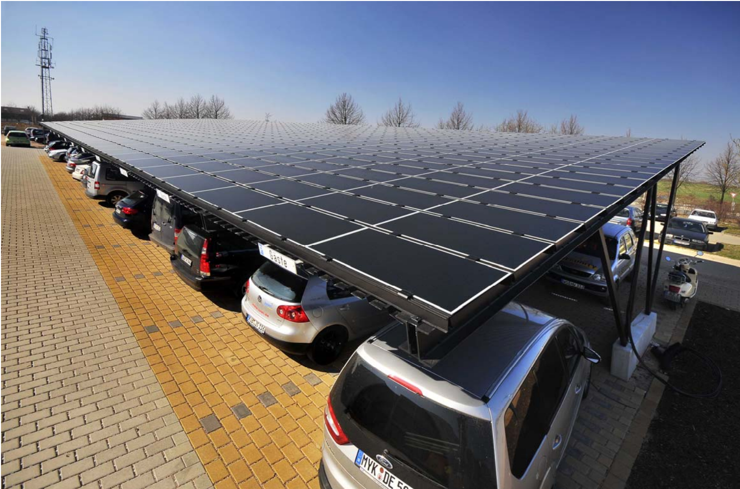
Carports at juwi's headquarters in Wörrstadt, Germany: 48 kWp (modules supplied by various manufacturers)
