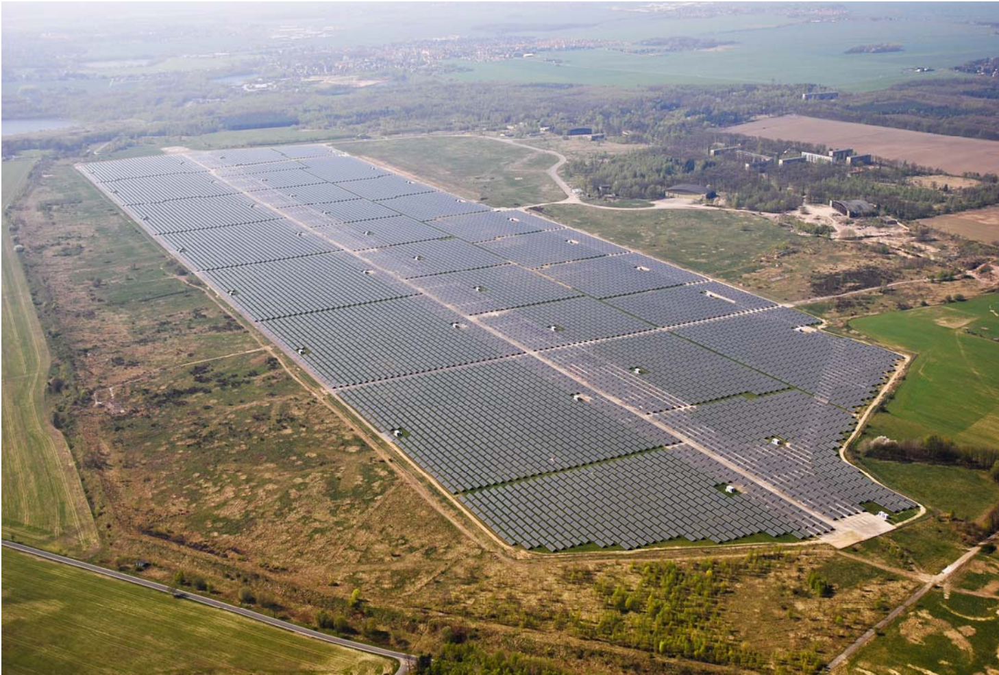
Former airfield in Brandis/Waldpolenz, Saxony: 40,000 kWp (modules supplied by First Solar)
