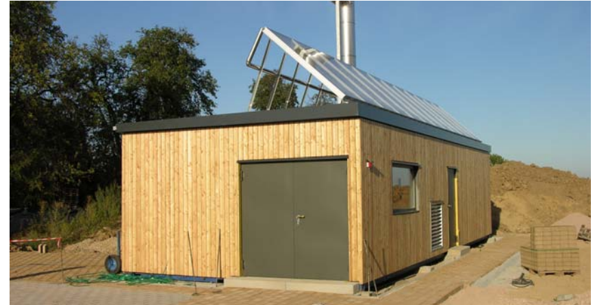
Energy cabin at juwi's headquarters in Wörrstadt
