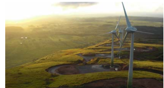
50-MW wind farm in Costa Rica
