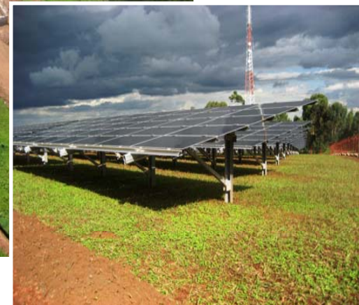
Mont Jali in Kigali, Rwanda: 250 kWp (modules supplied by First Solar)
