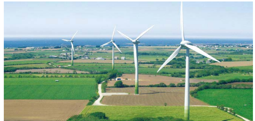
Wind farm in Brittany, France
