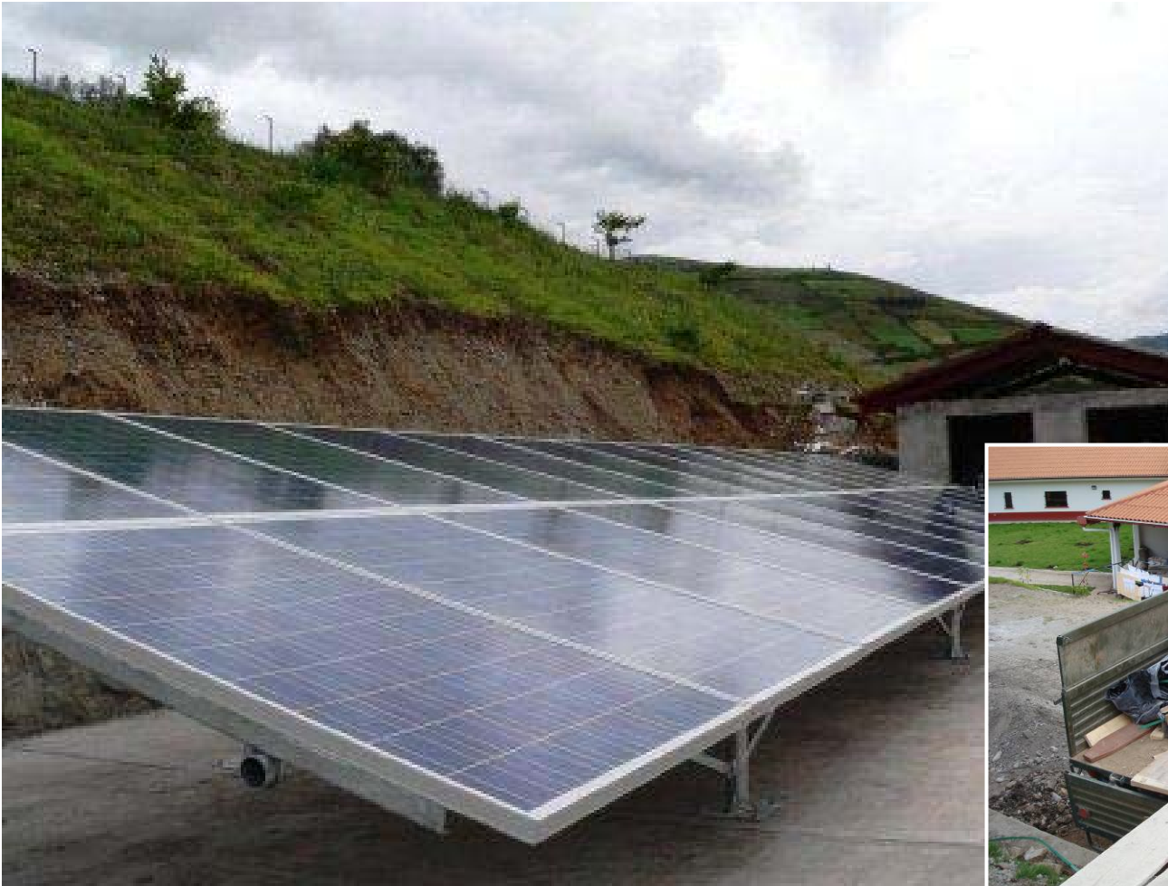
Power for the lightning system of a hospital in Peru 5.7 kWp + battery storage system
