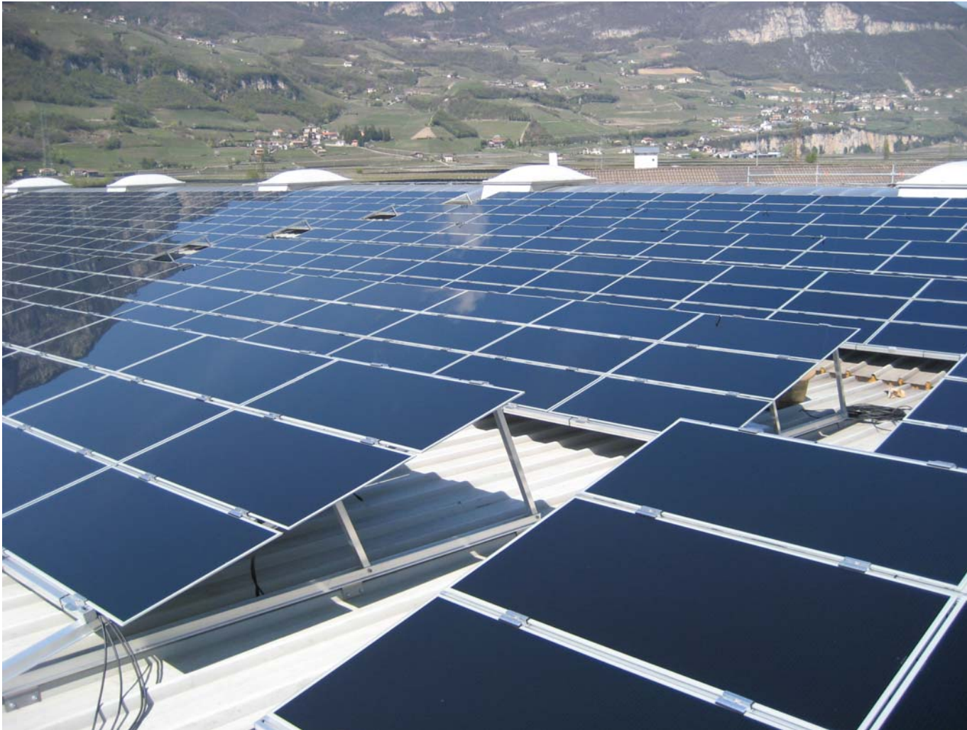
Market hall in South Tyrol, Italy: 520 kWp (modules supplied by First Solar)
