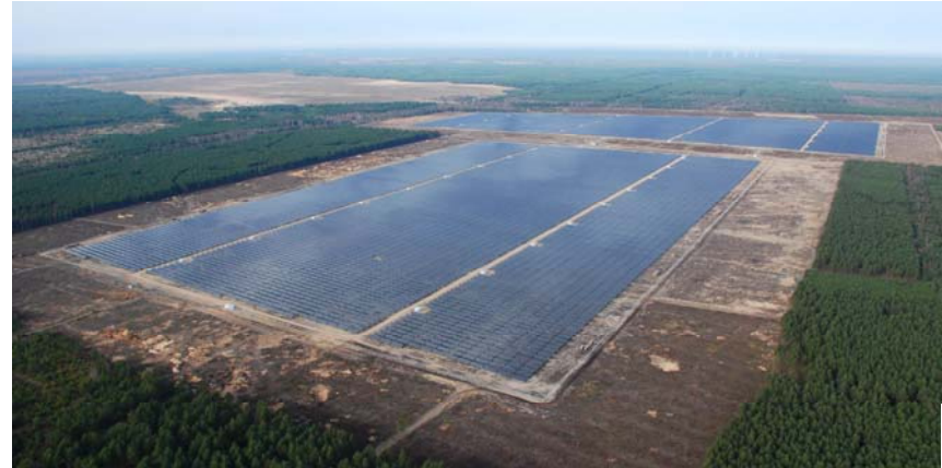
Free-field installation / former military area in Brandenburg, Germany
