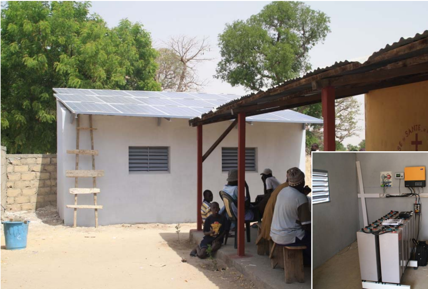
Power for a local hospital station in Senegal 3.96 kWp + battery storage system
