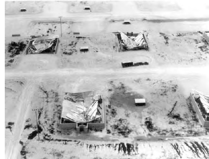
Ash fall and roof collapses during the 1992 eruption of Pinatubo, Philippines © USGS
