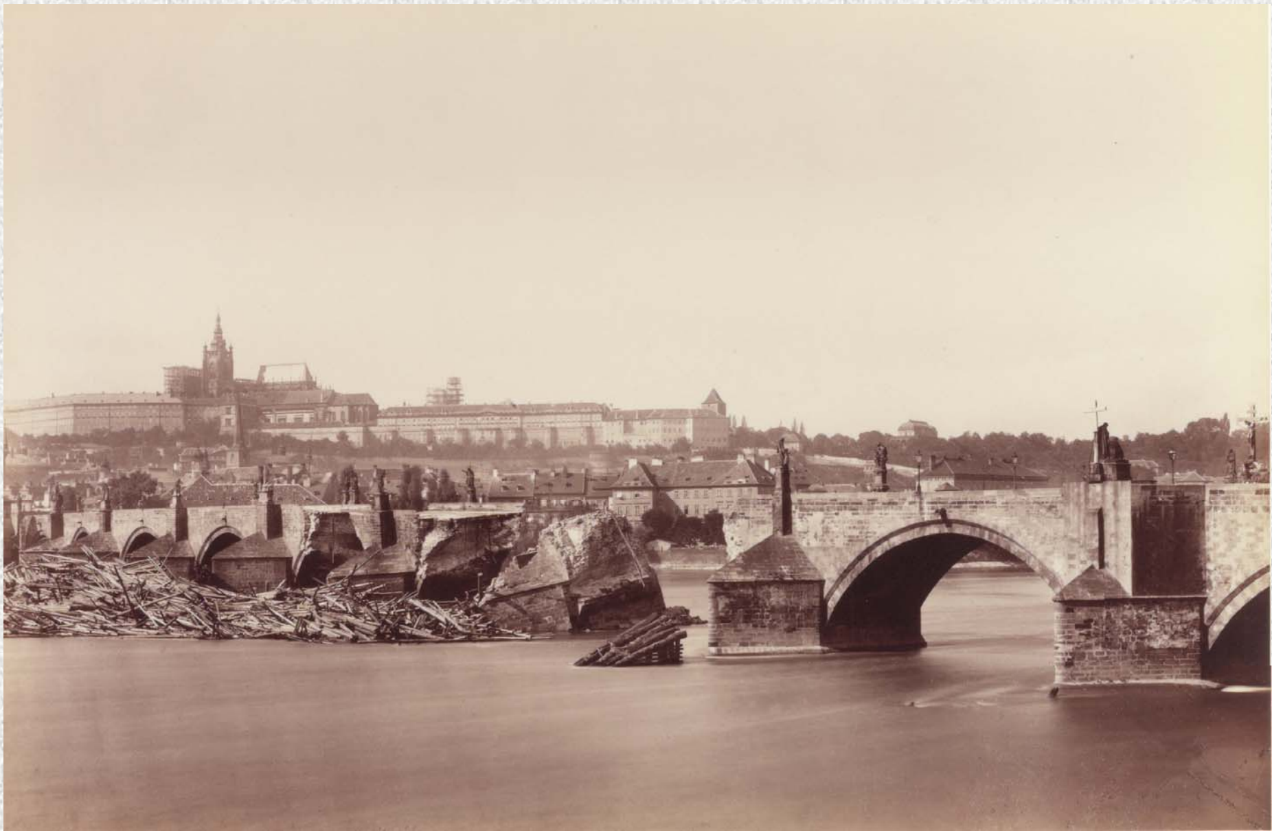
Damaged Charles Bridge in Prague after flood in September 1890
