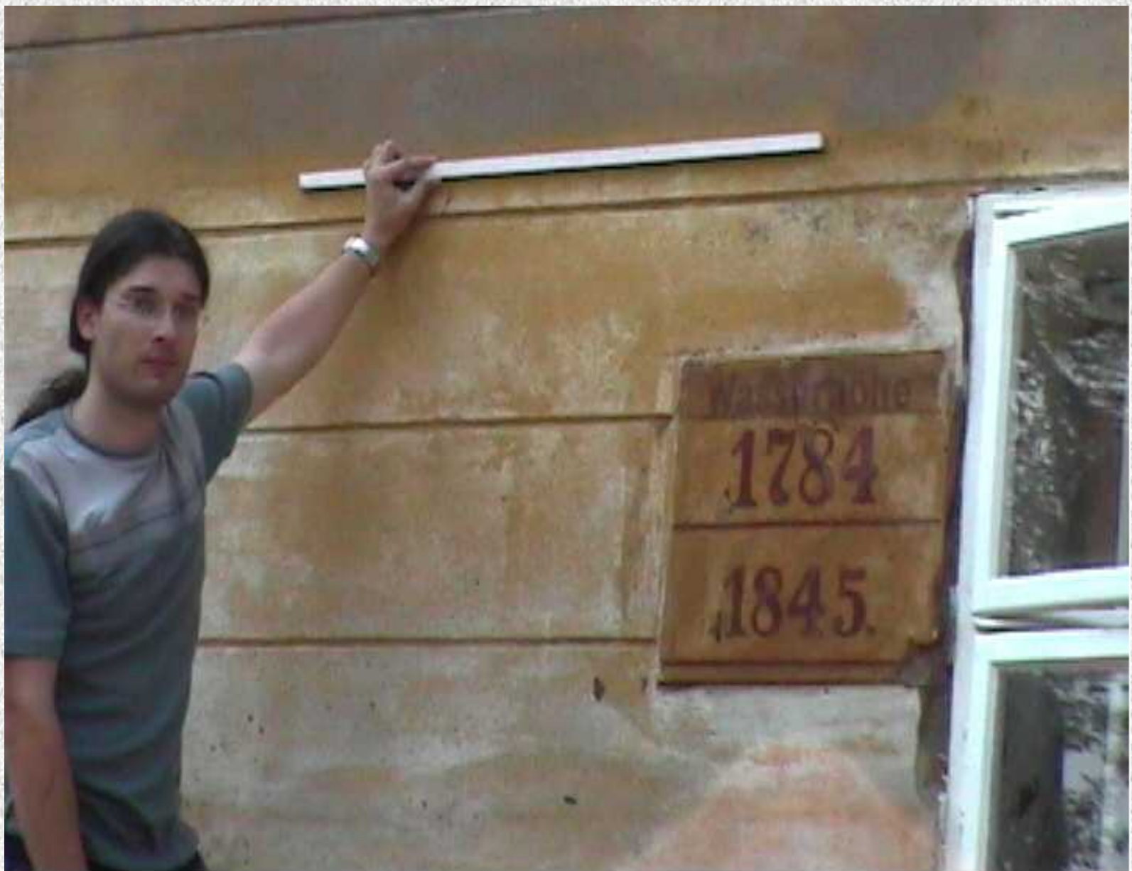
Watermarks at Kampa in Prague - comparison of the Vltava floods from 2002 (August), 1784 (February) and 1845 (March)
