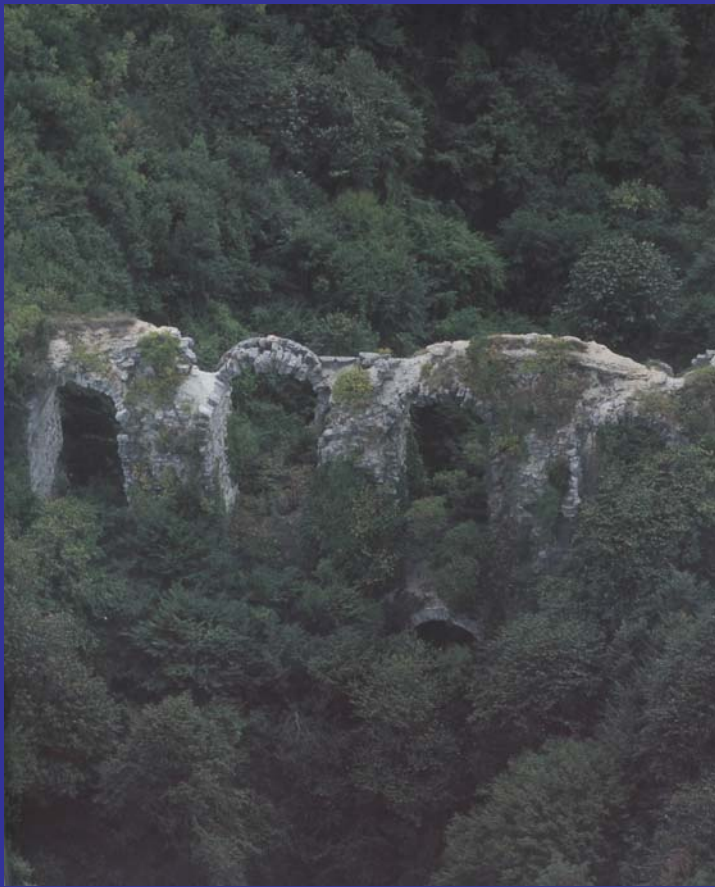
The Keçigerme Aquaduct System: one of the 40 along the way of the Strandja water supply system
