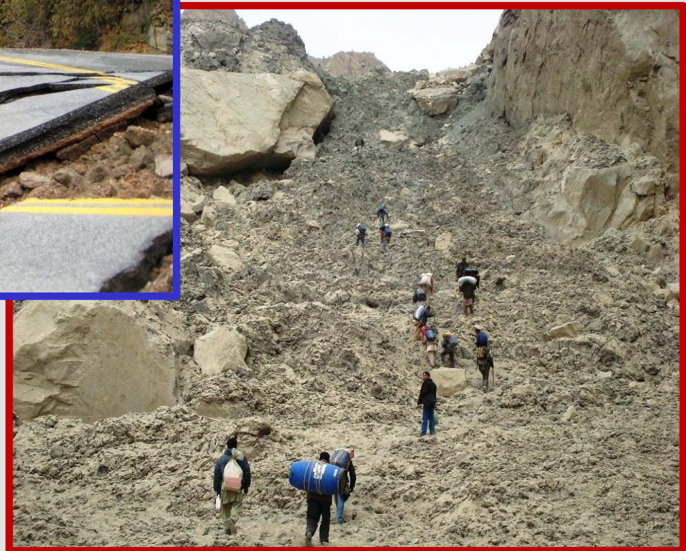
Attabad Landslide (Jan 2010), Karakoram Highway. (Image: Parnir Times, 2010)
