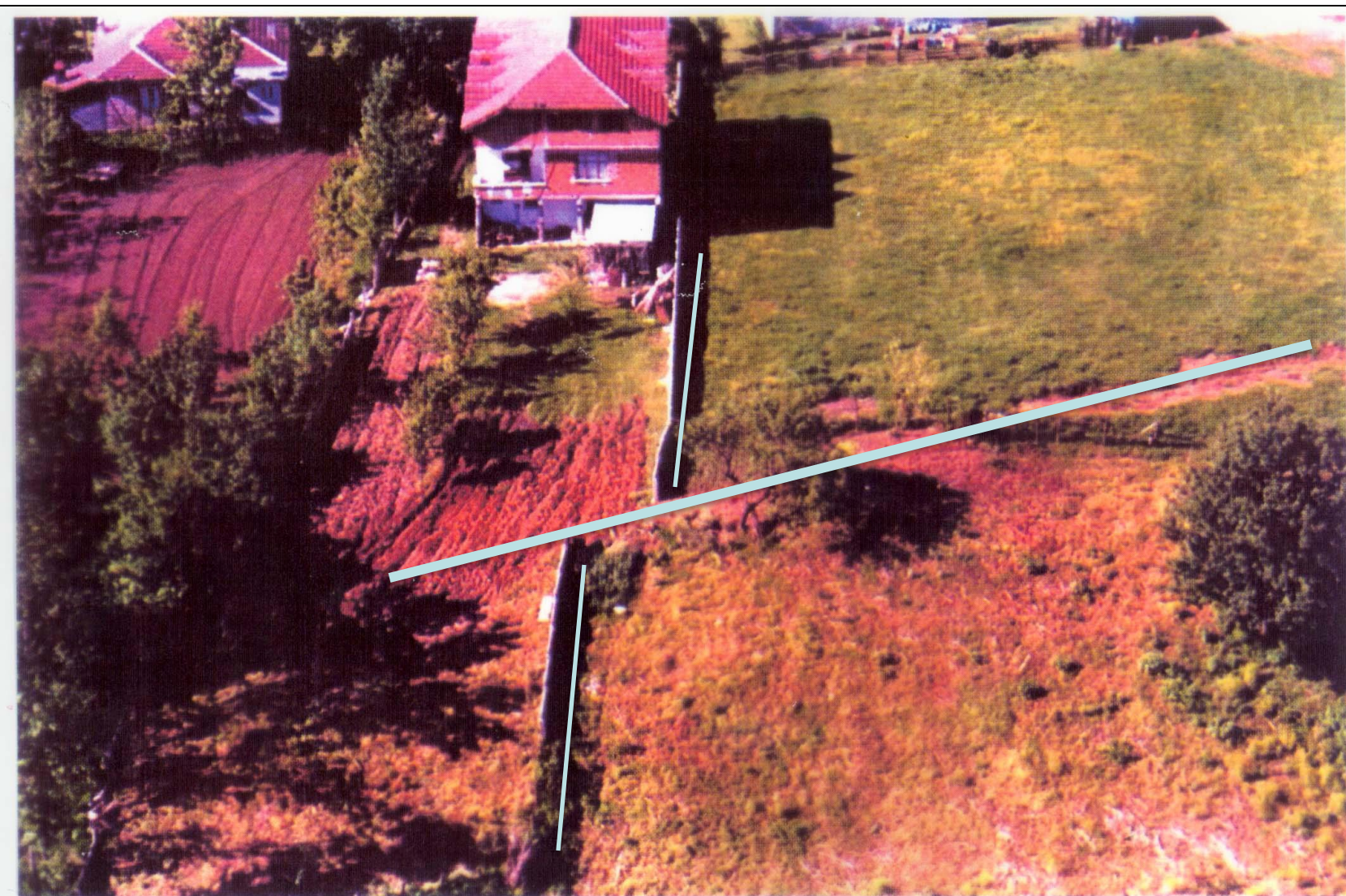
Figure 6. The 4.3 m offset of the garden wall near Çınarlı village, east of Eften lake.
