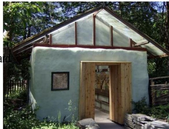
Straw bale building, Centre for Alternative Technology Machynlleth, Wales © ceridwen and licensed for reuse under this Creative Commons Licence
