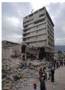
Damaged buildings in the Port-au-Prince neighbourhood of Haiti, after the 2010 Haiti earthquake. The tall block remains standing amid the ruins of lower, less well-constructed buildings. Photo by Marcello Casal Jr/AB, licensed under the Creative Commons Attribution 2.5 Brazil license.
