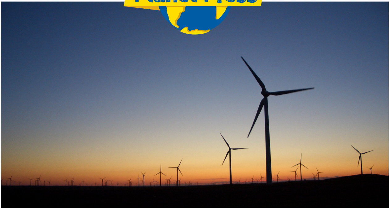
Large-scale wind power plant in China (Credit: Wenzhu Hou, distributed via imageo.egu.eu )
