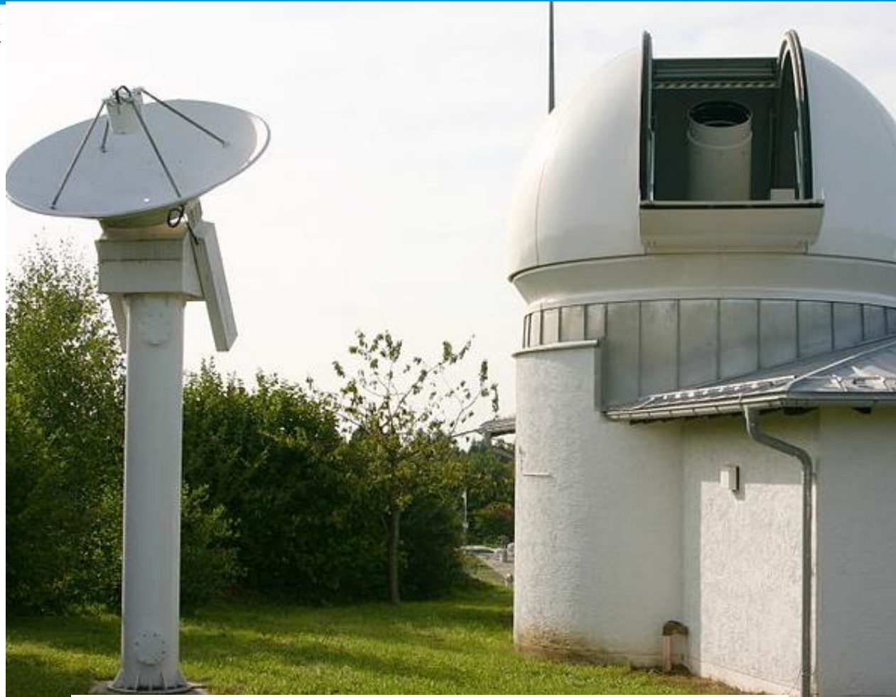
Laser Ranging System of the geodetic observatory Wettzell, Bavaria
