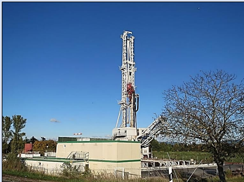
Hydrothermal power plant and borehole, Brühl, western Germany
