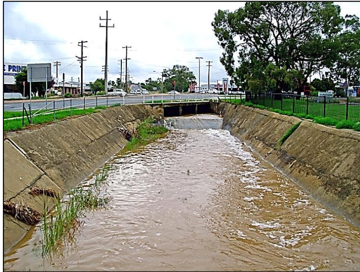
Figure 6.7. Storm drain, Dobney Avenue, Wagga Wagga, New South Wales, Australia
