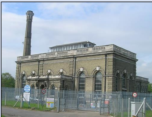
Victorian pumping station, London, England, that once contained a huge steam pumping engine
