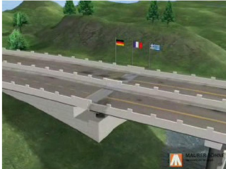
Expansion Joint: Device to accommodate tectonic movement, deck vibrations and any deck length variation
