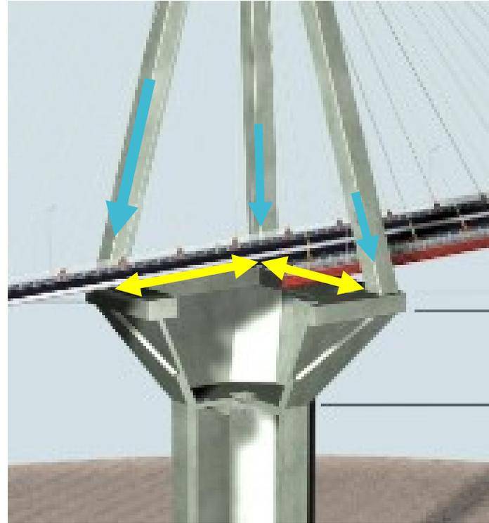
Square structure of high strength (C50/C60) pre-stressed concrete beams to rigidly connect pylon legs
