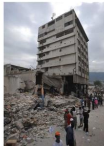
Damaged buildings in the Port-au-Prince neighbourhood of Haiti, after the 2010 Haiti earthquake. The tall block remains standing amid the ruins of lower, less well-constructed buildings. Photo by Marcello Casal Jr/AB, licensed under the Creative Commons Attribution 2.5 Brazil license.
