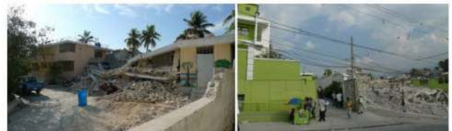
Figure 1a (left). Collapsed private school in central Port-au-Prince metropolitan region; a neighboring single-family house sustained no damage; (b, right) Well-built commercial building (left side) adjacent to catastrophic collapse of neighboring structure.
