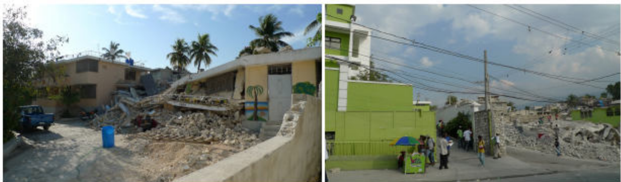
Figure 1a (left). Collapsed private school in central Port-au-Prince metropolitan region; a neighboring single-family house sustained no damage; (b, right) Well-built commercial building (left side) adjacent to catastrophic collapse of neighboring structure.
