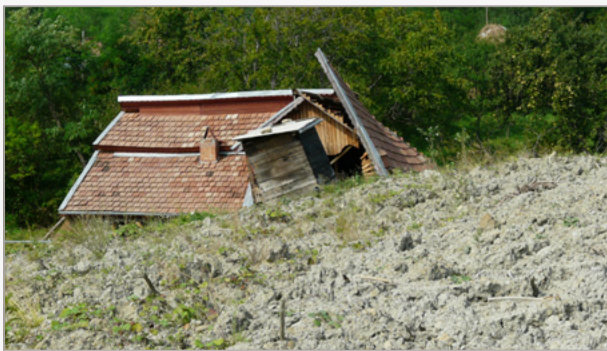
Natural hazards, such as landslides, often cause damage to human property and loss of lives. The picture shows a house damaged by a mud flow in the Buzau County, Romania. (Image distributed by EGU under a Creative Commons licence via www.imaggeo.net . Credit: Raluca-Mihaela Maftei)
